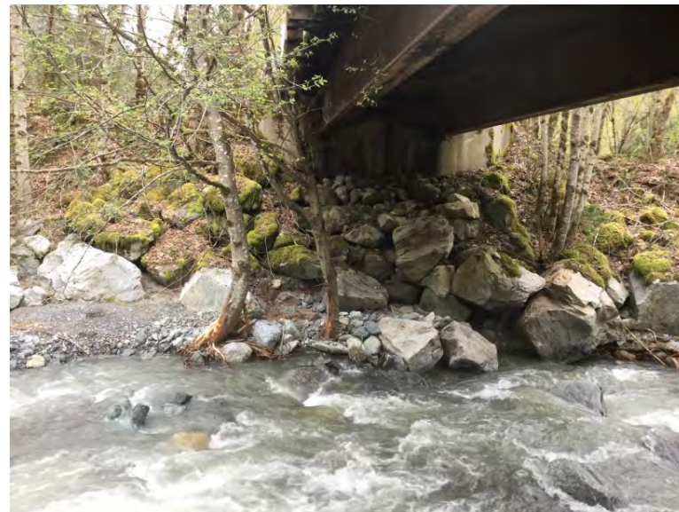
Left Bank Abutment when facing downstream
