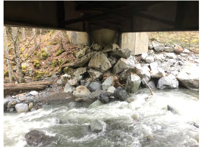
Right Bank Abutment when facing downstream
